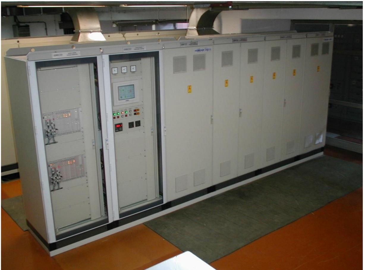
Figure 2 New Končar excitation system of the synchronous generator at Varaždin HPP, Croatia
